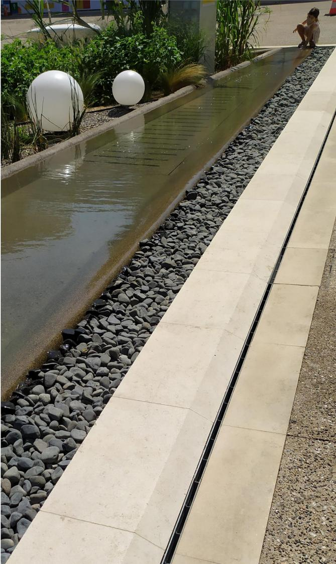
The drainage system with the Brickslot represents one of the possible types of water drainage and can be considered a valid alternative to the traditional gratings.
